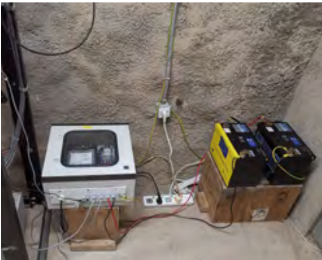
Corrective maintenance action at AS030 (Ethiopia) under EU funding.
