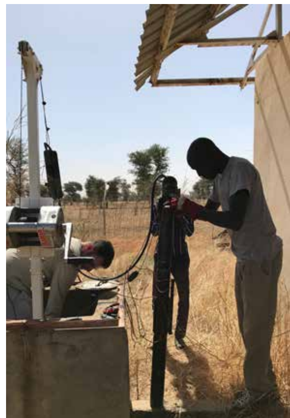
Changing the old borehole seismometer
