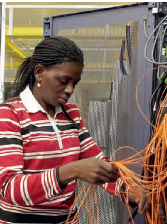
Left: laying optical fibre cables to integrate the database grid into the infrastructure of the storage area network. Right: servers in the computer centre.
