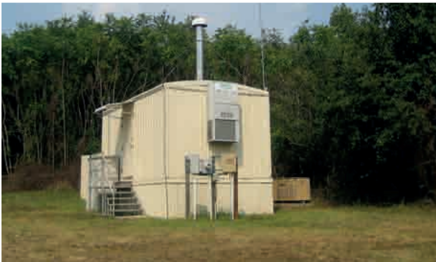
Above: radionuclide station RN68 on the island of Tristan da Cunha (United Kingdom) in the South Atlantic Ocean, whose noble gas measuring system was certified in December 2010. Below: radionuclide station RN75 at Charlottesville, Virginia, USA, whose noble gas system was the first to be certified as part of the IMS.
