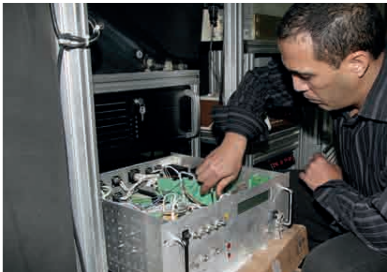
Above: lightning surge protection system installed at radionuclide station RN13, Edea, Cameroon.
