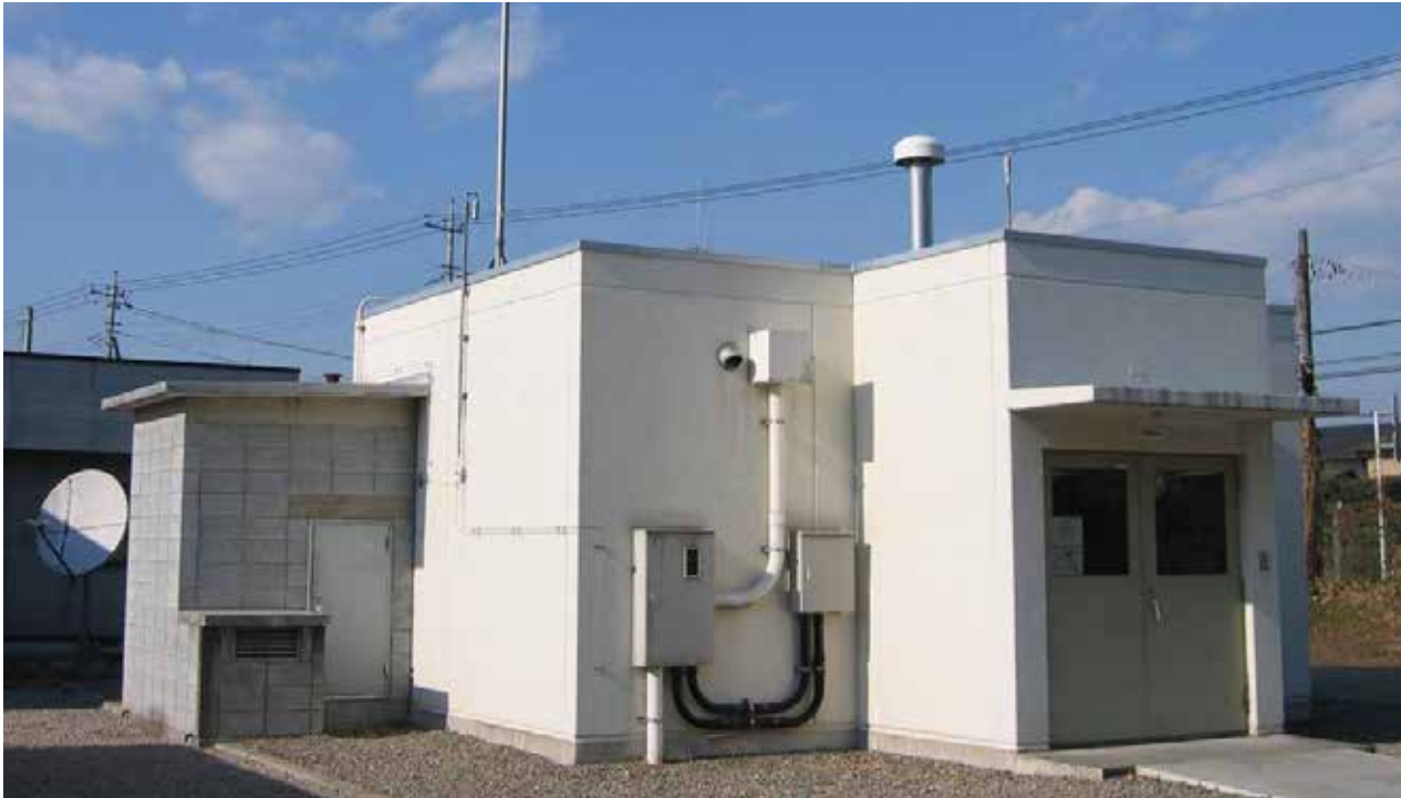
The certification of the noble gas monitoring system at radionuclide station RN38 in Takasaki, Japan, in December 2014 brought the total number of fully certified IMS facilities to 281. A further 19 stations have already been installed.
