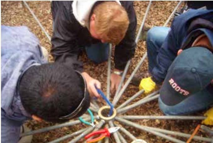
MAINTENANCE WORK AT IS14 JUAN FERNADEZ, CHILE
