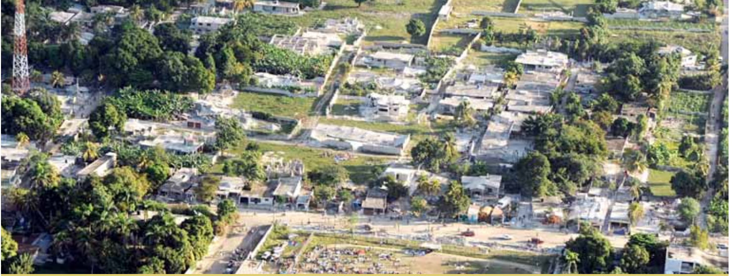
JANUARY 2010: Earthquake damage, Port au Prince, Haiti. Photo courtesy of U.S. Coast Guard Sandra Kay Kneen
