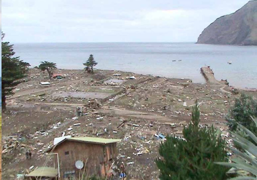
Juan Fernandez Island, Chile, showing the aftermath of the February 2010 tsunami. The IMS hydroacoustic station HA03 was destroyed by the tsunami.
