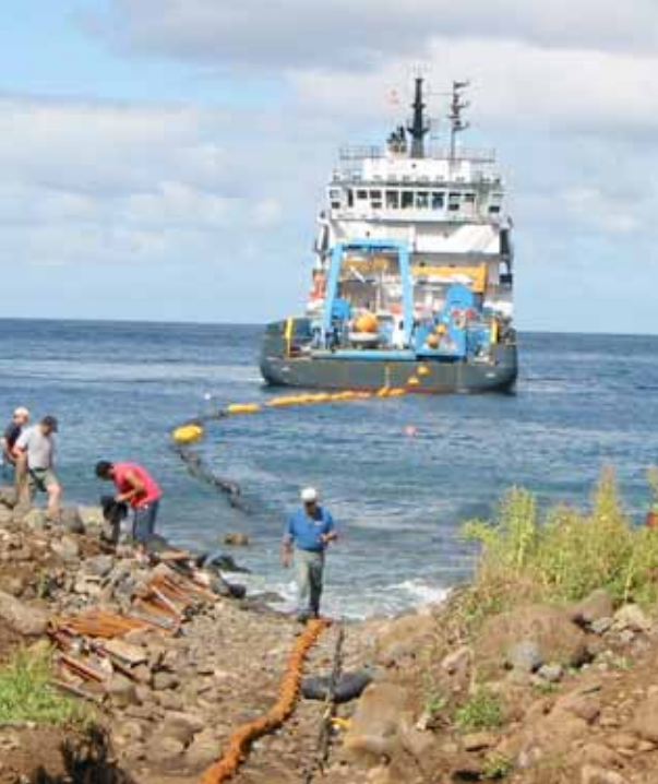
Installing the underwater cable of hydroacoustic station HA03, Juan Fernandez Island, Chile, in 2003.
