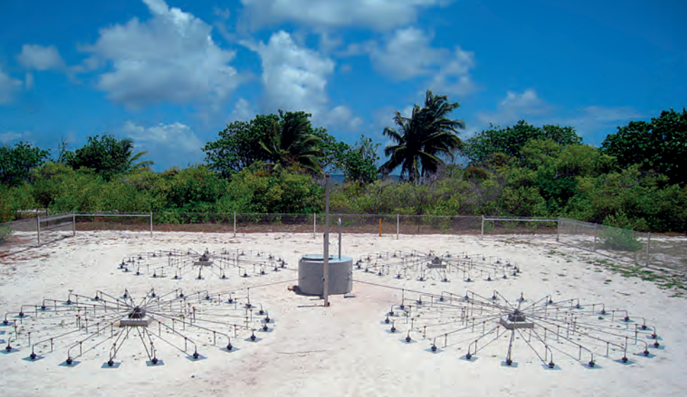
Infrasound station IS6 on West Island in the Cocos Islands (Australia) in the Indian Ocean, approximately midway between Australia and Sri Lanka.
