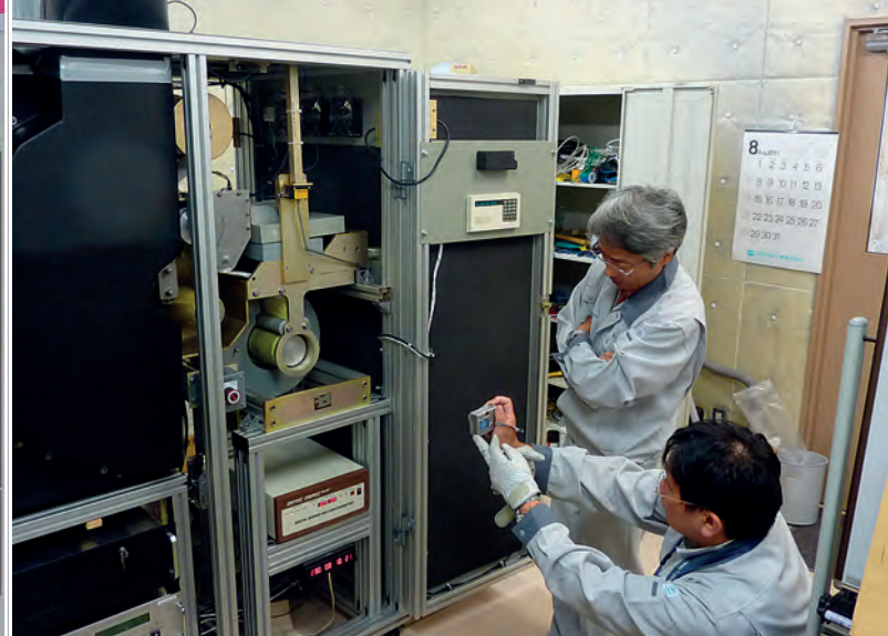
Operators verifying the installation of the detector system at RN38.
