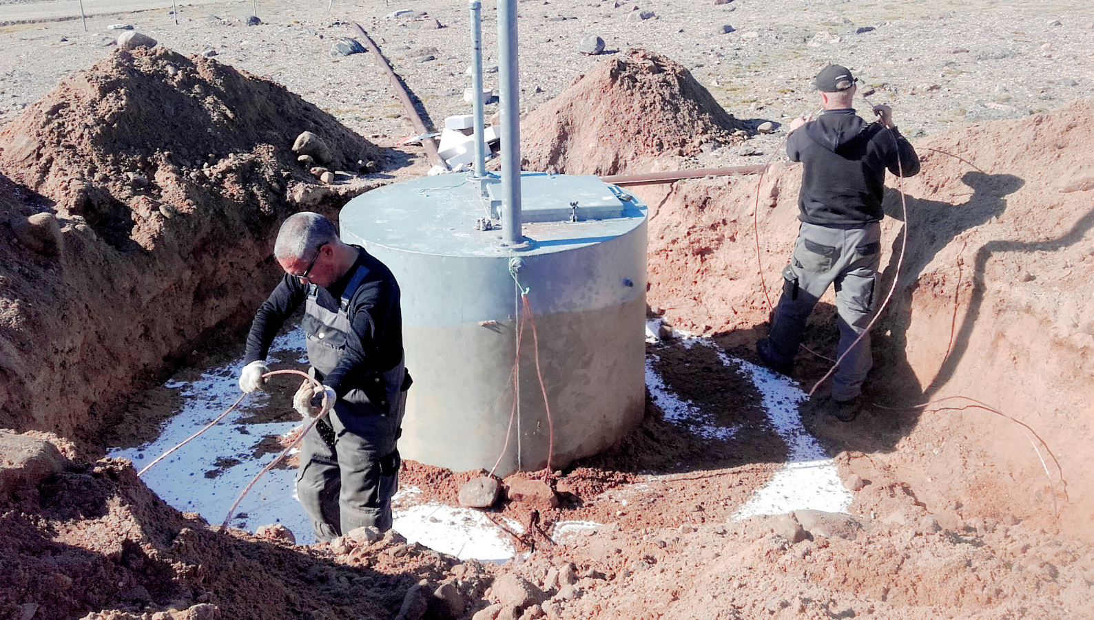
Station de surveillance des infrasons IS18, Qaanaaq, Groenland (Danemark).
