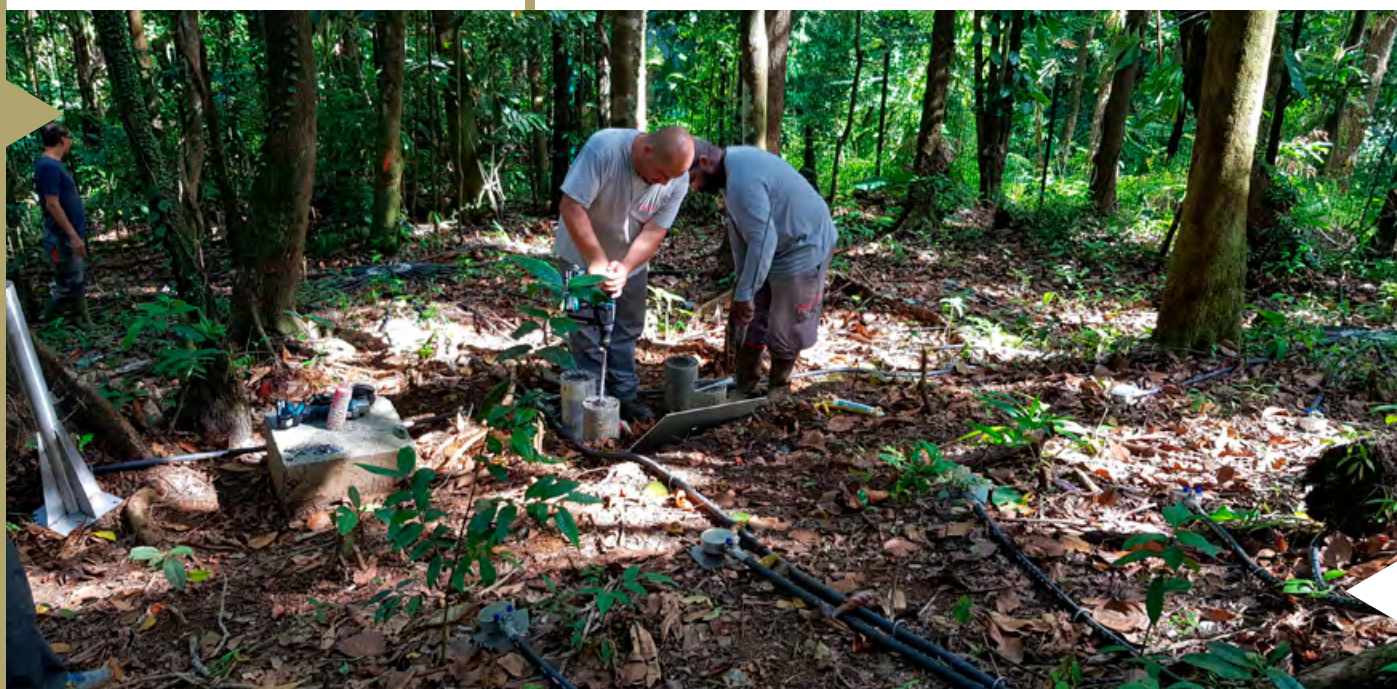
► Installation of Infrasound Station IS25, Guadeloupe, France.
