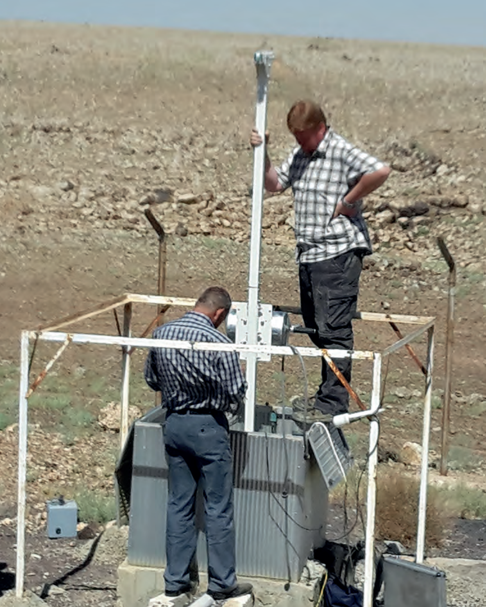
Sensor installation at auxiliary seismic station AS56, Tel-Alasfar (Jordan)
