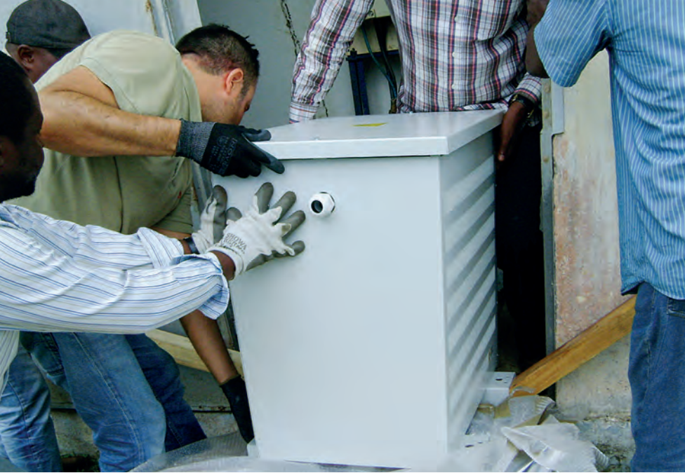
Installation of a new transformer at radionuclide station RN13, Edea (Cameroon)
