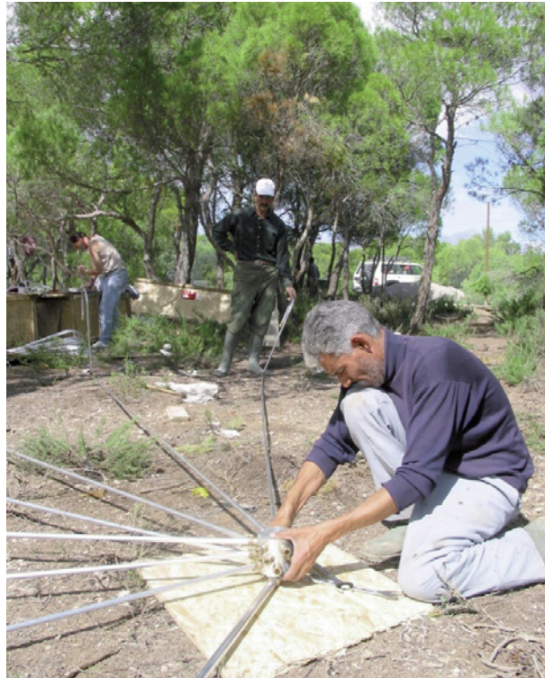
First installation of PTS-supplied prefabricated pipe array, infrasound station IS48, Kesra, Tunisia.
