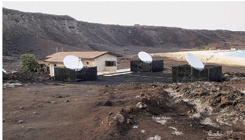
Central recording facility and satellite communications antennas at hydroacoustic station HA10, Ascension, United Kingdom.
