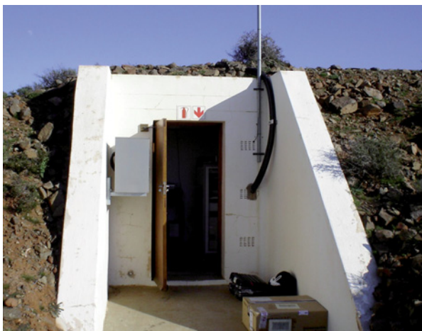
Vault entrance, auxiliary seismic station AS99, Sutherland, South Africa.
