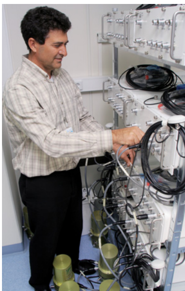
Preparation and testing of infrasound station equipment.
