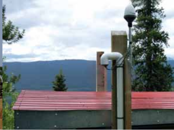
Antenna for Global Positioning System on vault of auxiliary seismic station AS13, Dease Lake, British Columbia, Canada.
