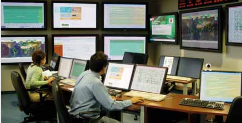
Control room of the Operations Centre.
