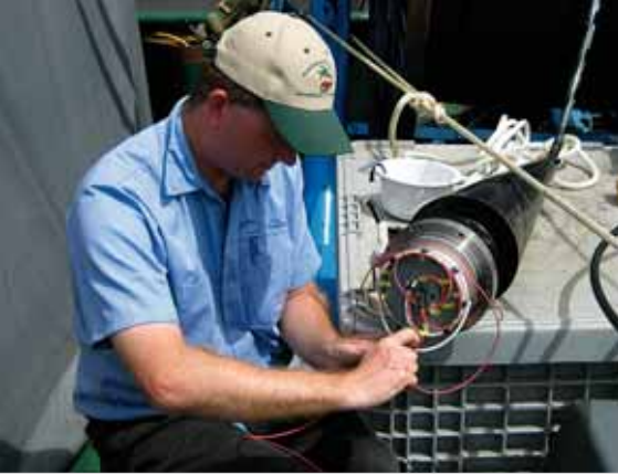
Above: Cable repair at hydroacoustic station HA3, Juan Fernández Island (Chile).
