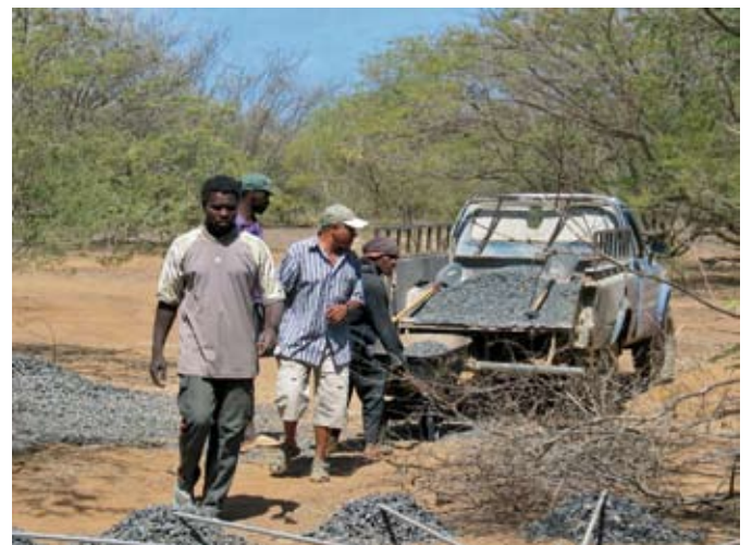
WORKERS PUTTING THE GRAVEL ON THE INLET PORTS, IS11, CAPE VERDE
