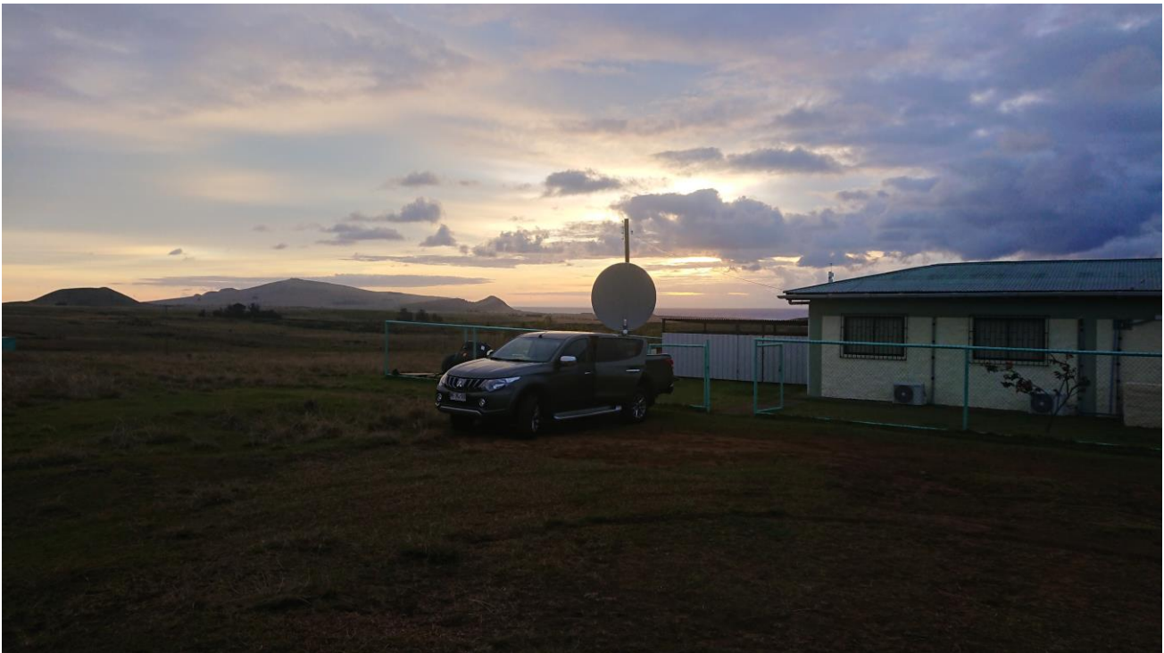
Figure 1 Station building, and generator shed.
