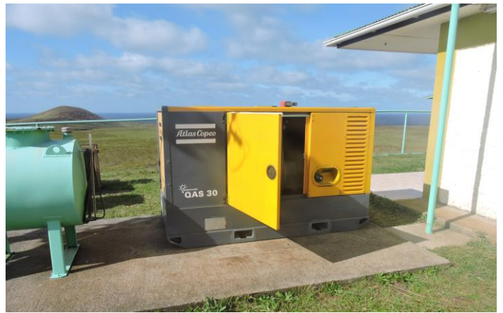
Figure 2 Existing generator and fuel tank on concrete base, front and back before the generator shed was constructed.
