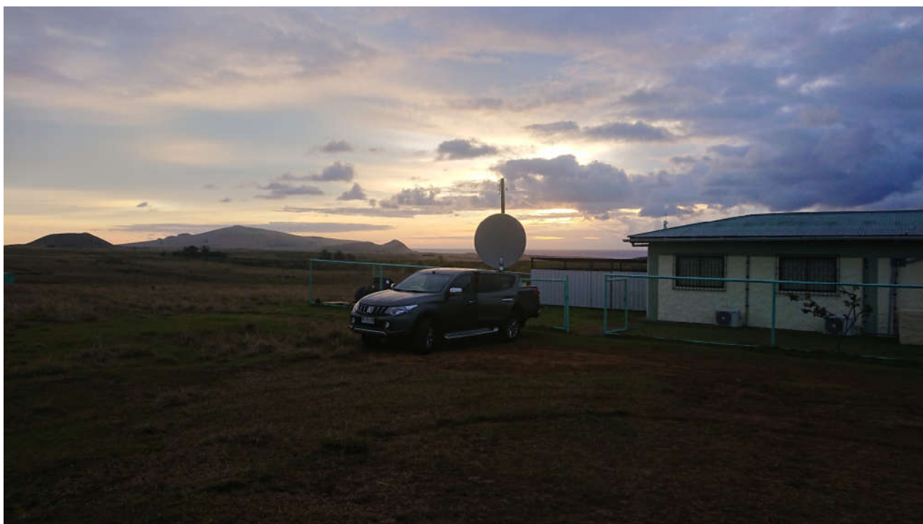
Figure 1 Station building and generator shed
