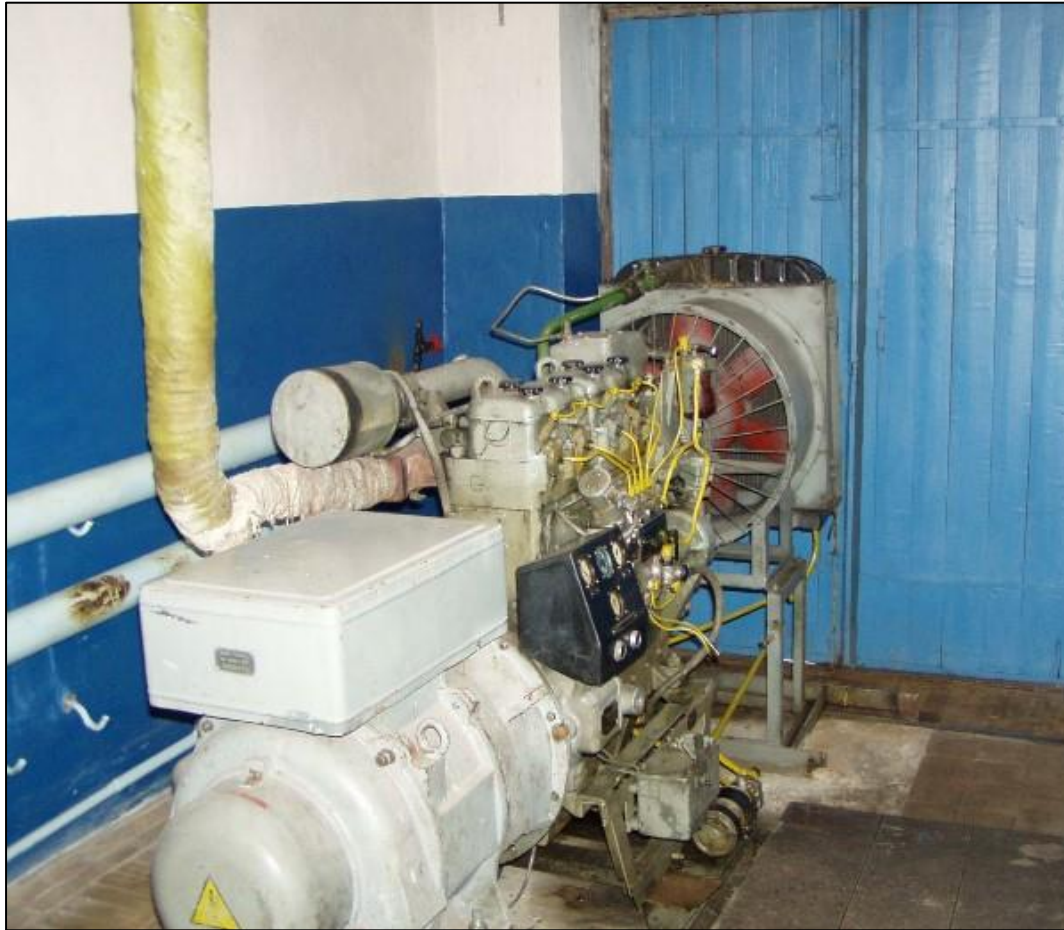
Left Photo: Diesel Generator ASDA2-20/T3400 (DG-1 20 kW) Right Photo Top: Diesel engine of Generator ASDA2-20/T400 (DG-1) Right Photo Bottom: Generator of 20 kW
