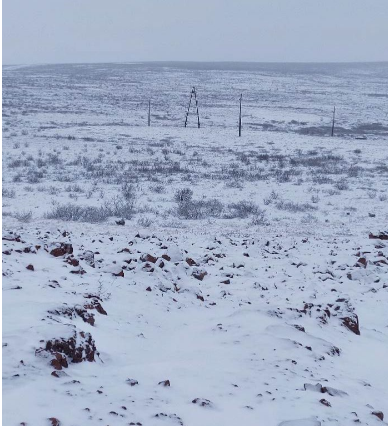
Figure 4. NRSK borehole site, view to the connection point of 6 kV line.
