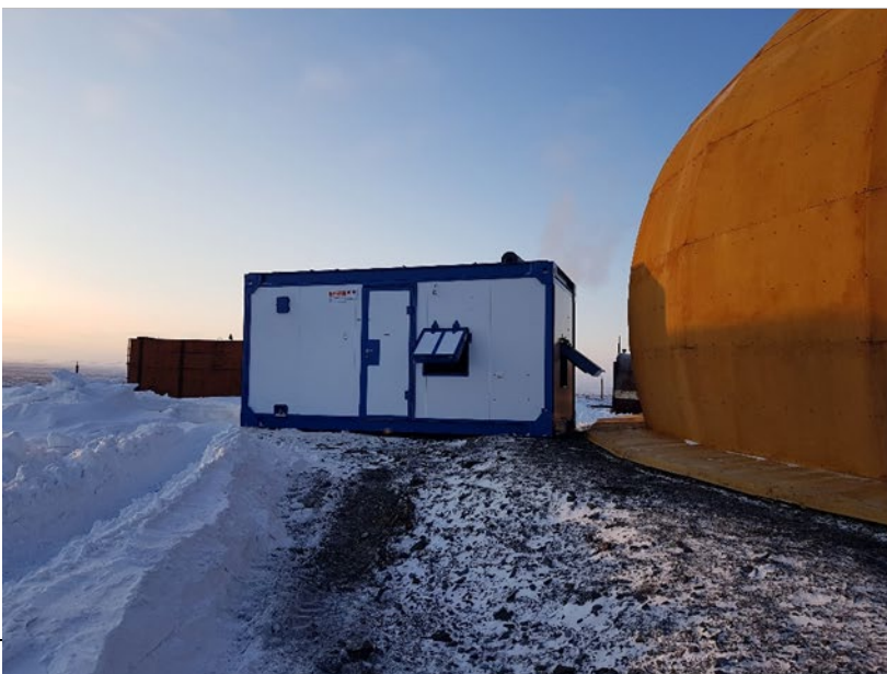
Design, Upgrade of Infrastructure and Logistic Support for relocation of IMS Primary Federation
