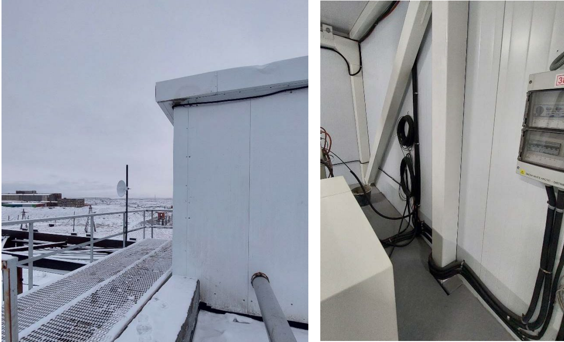
Figure 7. External and internal place for radio equipment on the roof of the CRF building.
