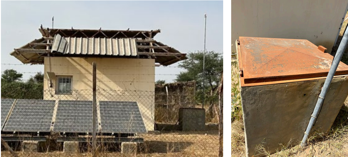
Fig 8.1 Overview with the borehole on the right of the building (left) and enclosure around wellhead (right)
