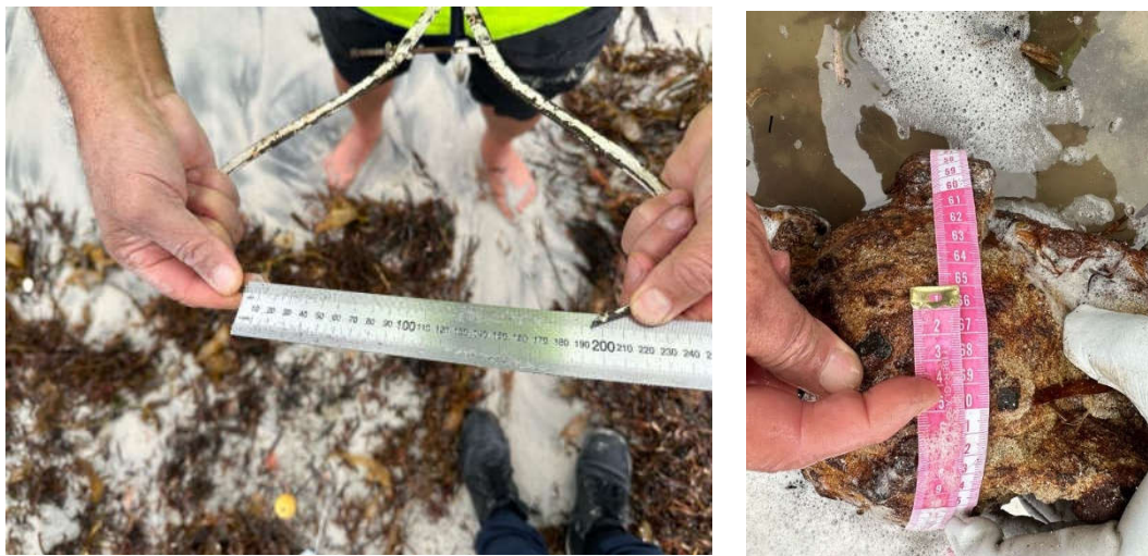
Figure B4: Measures of as-installed articulated split-pipe exposed on beach, to determine maximum outer diameter (May 2023) of 195 mm
