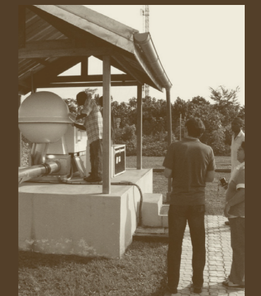
Installation of equipment at radionuclide station RN13, Edea, Cameroon
